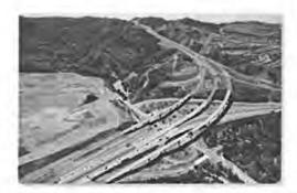
**Description:** The project consists of constructing a single lane tolled connector between the median of the SR 91 Express Lanes and the median of SR 241.
